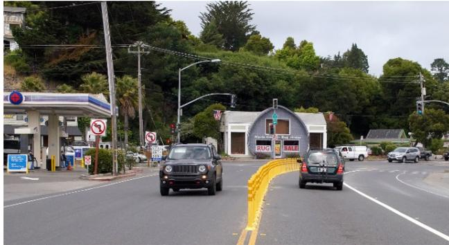
Construction activity for the Tam Junction Bicycle and Pedestrian Improvement project is expected to be complete by the end of February. Construction crews have relocated utilities, added a retaining wall and realigned curbs and sidewalks to make room for the pedestrian and bicycle facility improvements. Upcoming activity includes relocating existing traffic delineators, installing traffic signal detectors and restriping the roadway with the new bike lanes.
